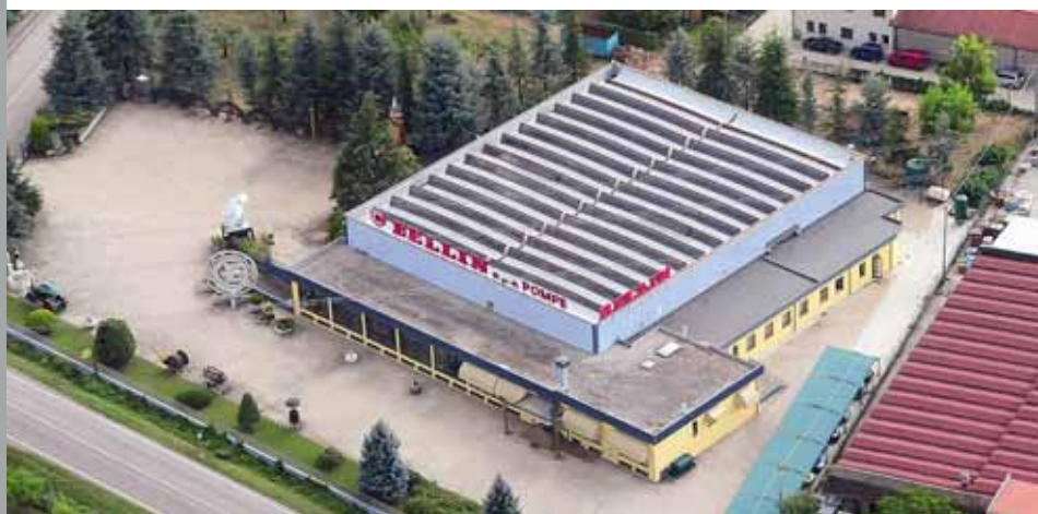
HEADQUARTERS - PRODUCTION UNIT 2
