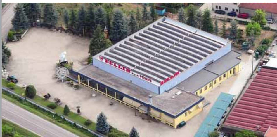
HEADQUARTERS - PRODUCTION UNIT 2
